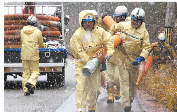
Training for laying makeshift conduit from Otsubogawa Dam
