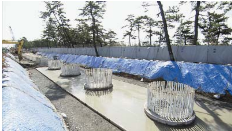
[Construction of tide embankment]
