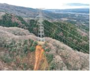
Collapse of ground and mountain surfaces around 275 kV transmission towers
