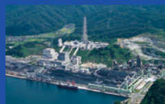
Tsuruga Thermal Power Station Unit 1
