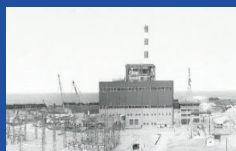
Toyama Thermal Power Station Unit 1
