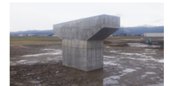
Example of Use in Public Works (Bridge Pier)
