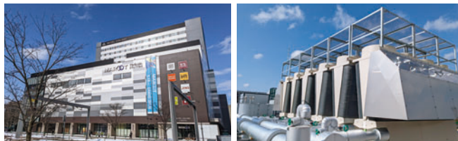
Maroot Air Conditioning Equipment (Heat Pump Chiller)
