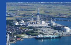
LNG-fired Unit 1 of Toyama Shinko Thermal Power Station
