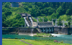
Jinzu River No. 1 Power Station (Hydro Power)
