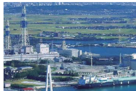
2018: LNG-fired Unit 1 of Toyama Shinko Thermal Power Station commenced commercial operation
