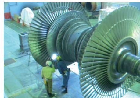
Regular inspection of a thermal power station
