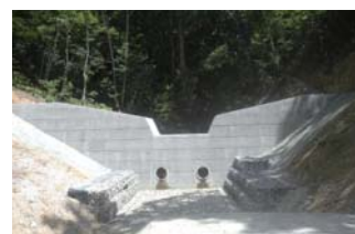
Erosion control dam
