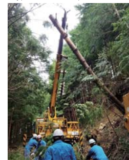
Disposal of fallen trees and removal of damaged equipment
