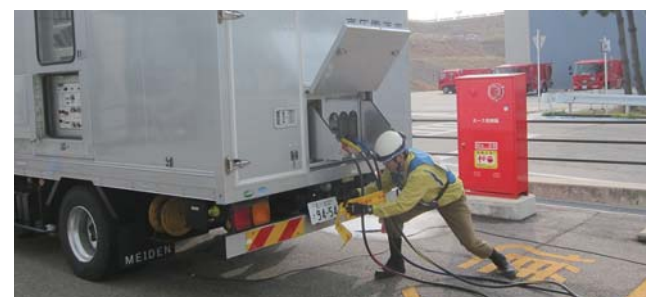
Power Supply Training with High-Voltage Power Supply Vehicles
