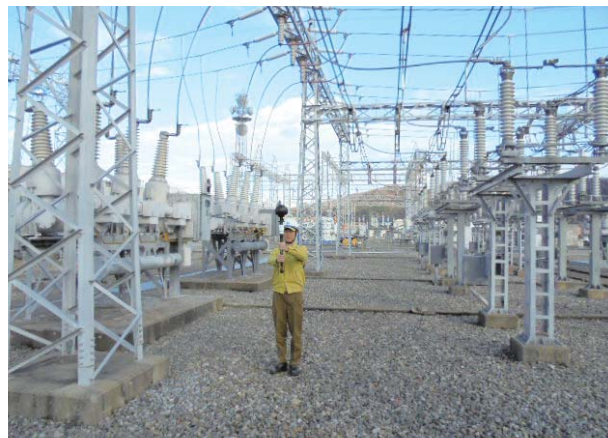
Streamlining through the use of new technologies (field survey using 360° camera)
