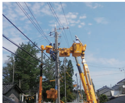
Concrete Pole Replacement Work
