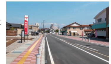
Townscape after Removing Electric Poles (Terai-machi, Nomi City)
