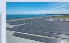
Mikuni Photovoltaic Power Station
