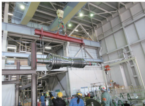
Replacement of All Turbines at Nanao Ohta Thermal Power Station Unit 1
