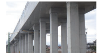
Elevated Hokuriku Shinkansen Line
