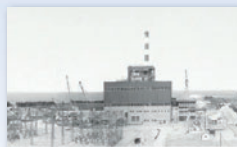
Toyama Thermal Power Station Unit 1
