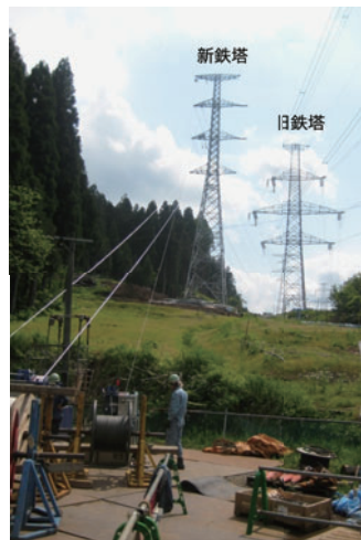
Transmission Tower Construction Work
