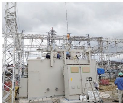
Transformer Replacement Work
