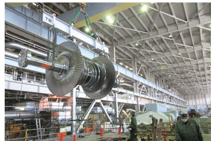
Replacement of the Turbine during Periodic Inspection of Nanao Ohta Thermal Power Station Unit 2
