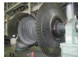
Regular inspection of a thermal power station
