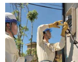
Smart meter installation
