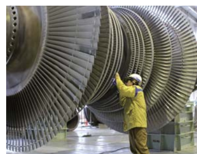
Periodic Inspection at Thermal Power Station
