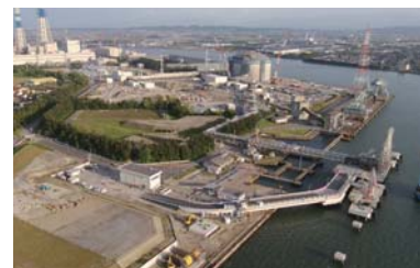
Overall view of the LNG facilities
