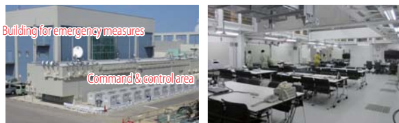
Exterior of command & control addition
