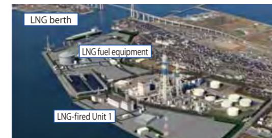
Image diagram of LNG-fired Unit 1 of Toyama Shinko Thermal Power Station
