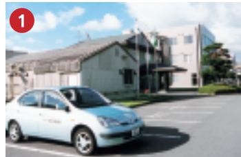
1 TANAKA CHEMICAL CORPORATION Factory to manufacture battery electrode materials at Technoport Fukui (Fukui)
