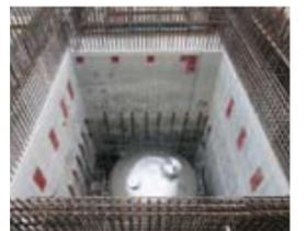
Situation of filtered vent equipment installation at Unit 2 (as of the end of July, 2015)
