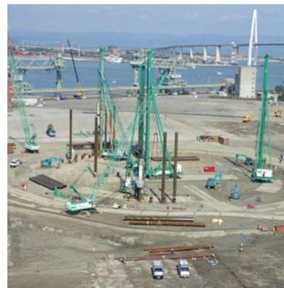
Placement of foundation piles for LNG tank
