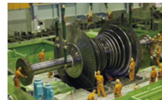
▲ Replacement with new rotor (low-pressure turbine rotor)
