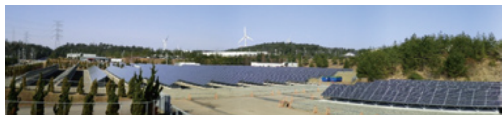
◀ Shika Photovoltaic Power Station
