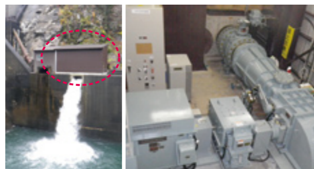
▲ Hotokebara Dam Power Station (right: inside the power station)
