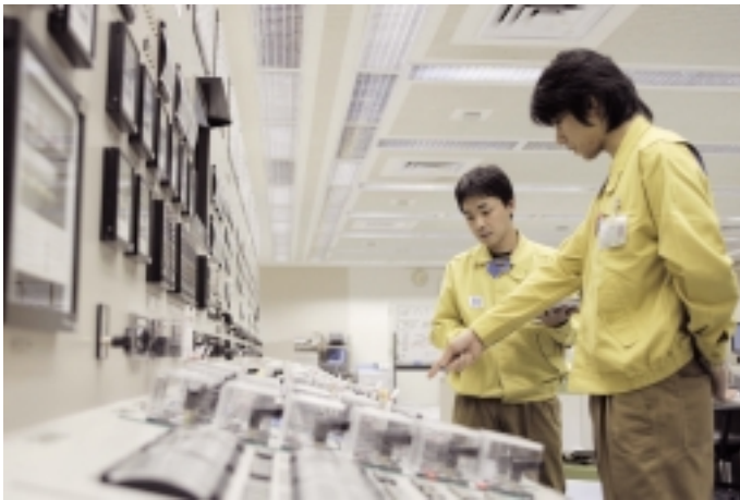
▲Technical guidance at nuclear power department
