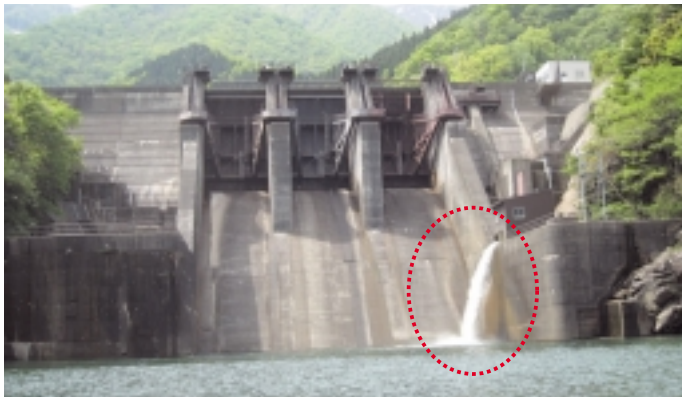
▲ Appearance of river maintenance discharge (Hotokebara Dam)
